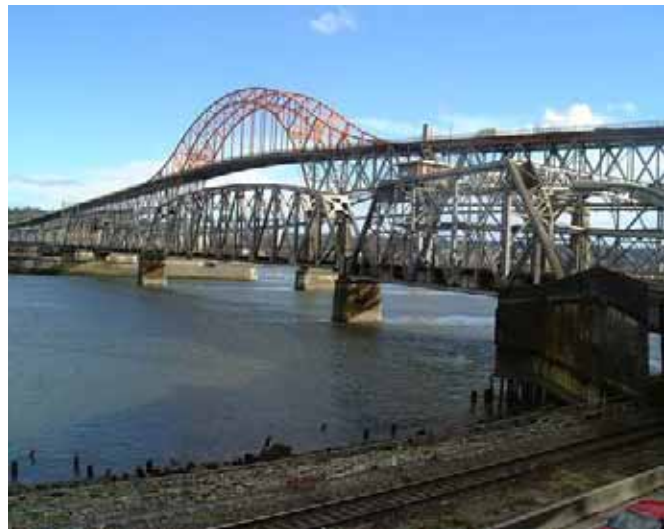
The New Westminster rail bridge (foreground) is at a low level and must be opened frequently for marine traffic. The Patullo highway bridge (immediately behind) and the SkyTrain bridge (background) were constructed high enough above the water to allow marine traffic to pass unobstructed.
