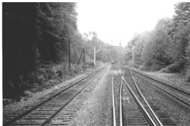
A crossover allows trains to change tracks.
