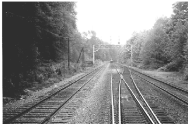
A crossover allows trains to change tracks.
