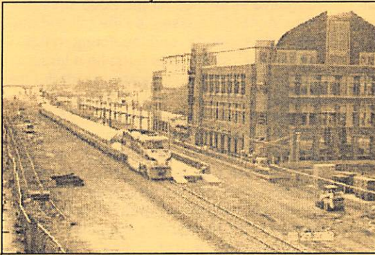
Amtrak Cascades train 761 passes the Everett Transportation Center on it's way to the Bond St. station stop. The train is adjacent to the new Amtrak platform that's finally under construction. Sound Transit was originally to build the platform as well as its Sounder platform and spur tracks. But BNSF and ST have yet to reach an agreement on ST's use of the BNSF right-of-way. Amtrak finally obtained right-of-entry from BNSF and signed it over to the city so that construction could begin. Amtrak expects to move its operations to the new station before the end of October. Photo by Warren Yee
