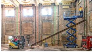
Workers hoist a steel beam that will be used to reinforce the wall. A winch on the second floor pulls the beam up and into place.
